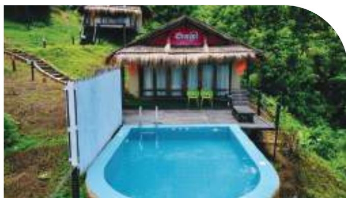
► The First Swimming Pool On the Ground Of sajek, Meghpolli Resort. Size: 10/15 feet
