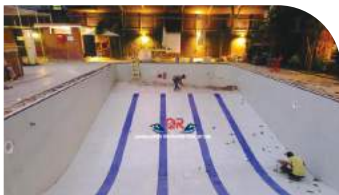
► Renovation Work at British Club. British High Commission Dhaka Baridhara
